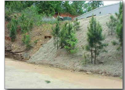
Figure 4. Slope covered with floc collection matting
