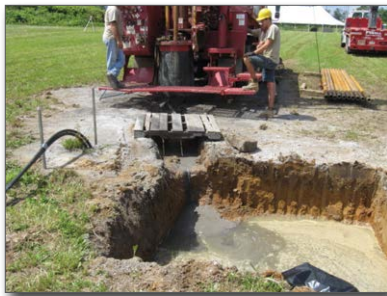
Figure 7. Drilling rig and settling pit
