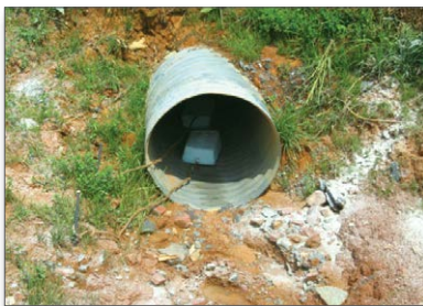
Figure 39. Polymer block in a construction site culvert
