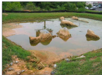
Figure 41. Same pond after BMPs were installed
