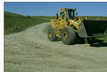
Figure 13. Road dust after applying polymer flocculant
