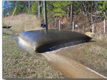
Figure 34. Sediment bag and its treatment ditch
