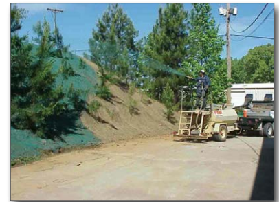
Figure 5. Hydroseeding the slope
