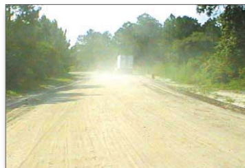
Figure 12. Road dust before applying polymer flocculant
