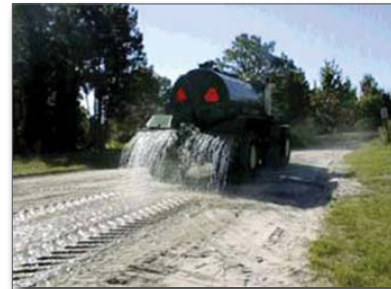
Figure 11. Water truck applying dissolved polymer flocculant
