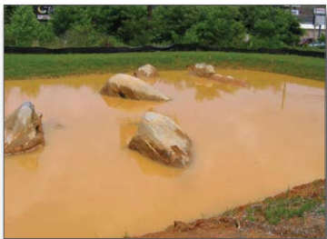
Figure 40. Sediment pond before BMPs were installed
