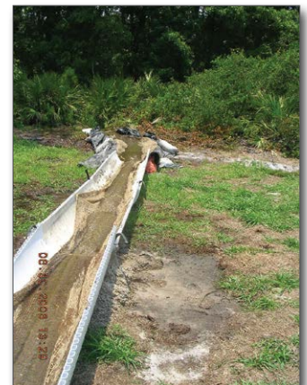
Figure 21. Split pipe with soft matting
