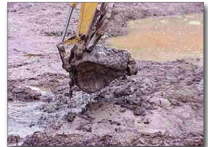
Figure 36. Removing stiffened sediment from a sediment basin
